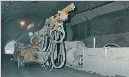
Tunnel Kirchdorf, mobile unit for asbestos
