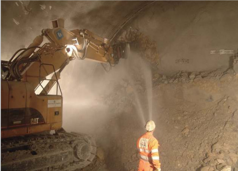
Cutter head, cutting process
