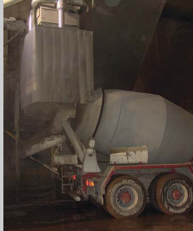
Loading of concrete mixing truck
