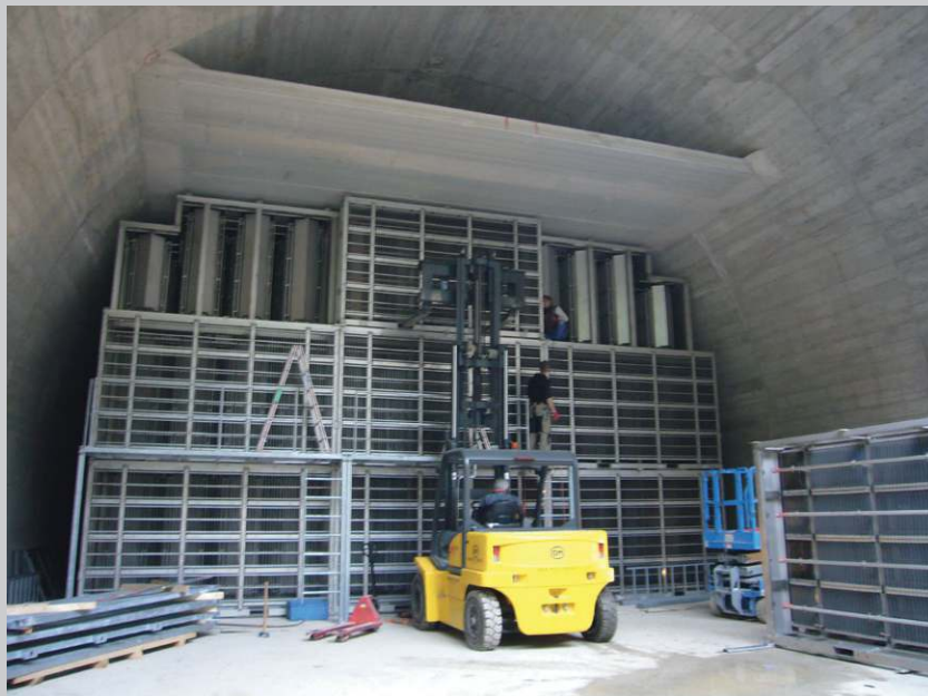
Installation of ECCO filter
