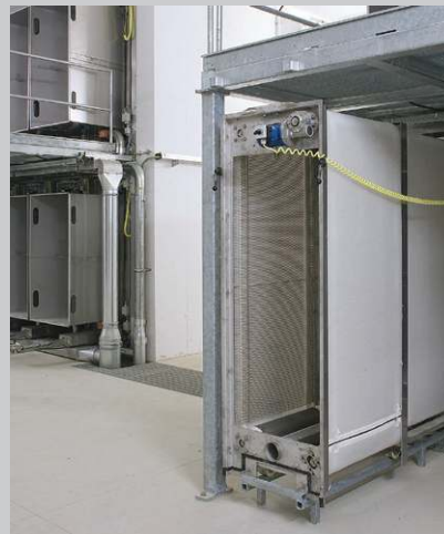
ECCO with dry cleaning system of collector
