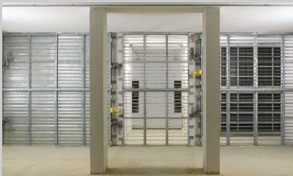
By-Pass with automatic dampers
